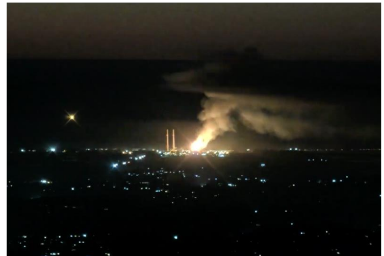
Arial night picture, Moss Landing Powerplant, battery storage fire, CA, USA, Jan. 16, 2025; 100,000 ft 2 storage building burned for 5-days.
